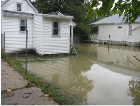
Flooding in Camden County after a typical rain event
